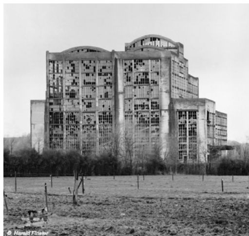
Fig. 3: Coal dressing plant "Lavoir Triage de Péronnes", 1-11-1993, by Harald Finster.
